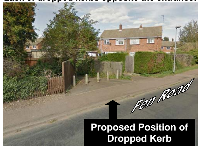
Photo 2 – Lack of dropped kerbs opposite the entrance:
